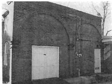
3. Toolhouse/Comfort Building: Built in 1887 it housed equipment, storage and toilets. The building originally extended to three bays, each reflected in a blind arch on the north wall. In 1927 it was connected to the lodge by a new wing. In 1952 the westernmost toolhouse bay was removed and the garage added. Today it is a utility building and maintenance shed.
