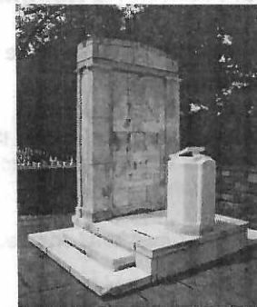
6. Rostrum: This 1945 marble rostrum replaced the original brick and wrought-iron rostrum from 1890. Although based on a standard plan from 1944, this is thought to be the only example of "Standard Rostrum Type A" built in the national cemetery system.
